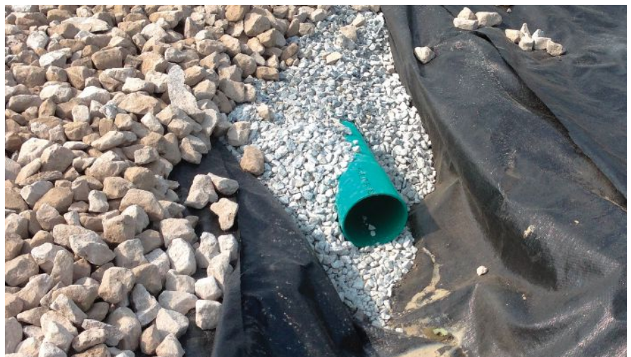
Top: Placing the Eco-Optiloc pavers; Bottom: Aggregate base and perforated pipe
